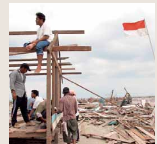
Rebuilding a mosque destroyed by the tsunami in Indonesia
